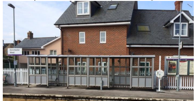
and the new shelter completed in April 2015
